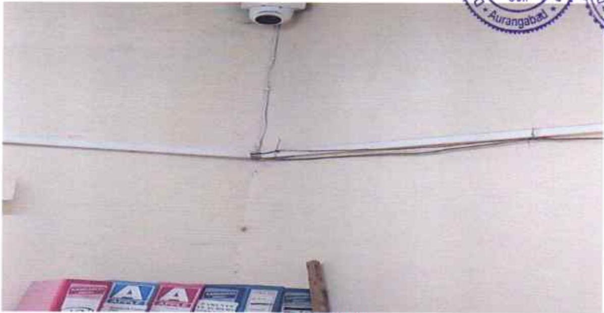
Camera inside Office
